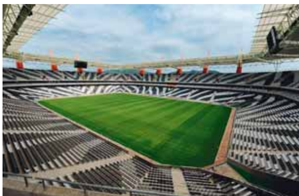
Nelspruit: Mbombela Stadium
